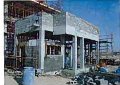
Lintel beams completed in Guard House
