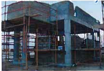
Block masonry in progress at Guard House
